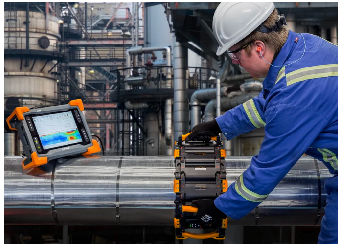
Figure 4: Lyft PECA pipeline CUI.
