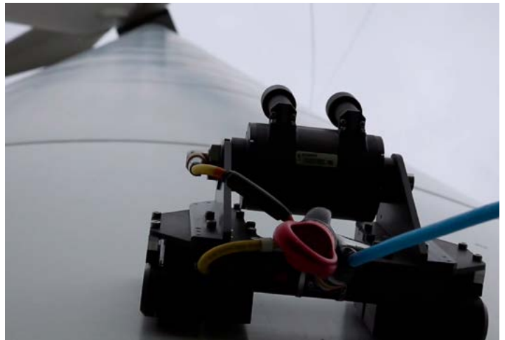
Remote visual inspection of a wind turbine
