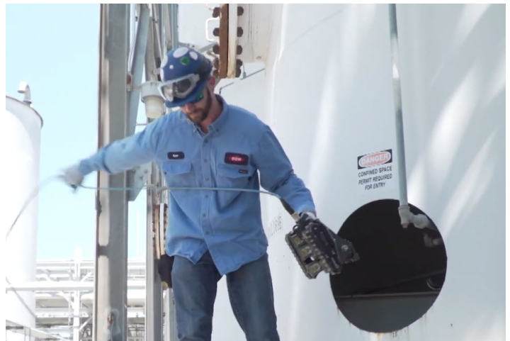
Confined space inspection
