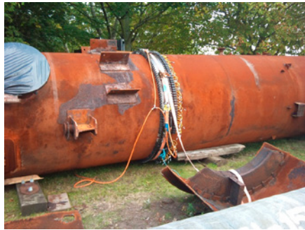
Figure 1. Teletest Focus guided wave ultrasonic test equipment applied to inspect the 66" vessel
