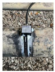
Figure 3: matPIMS™ 3×5 matrix permanently installed with RS-485 cable back to surface for data collection, pre-overwrap.
